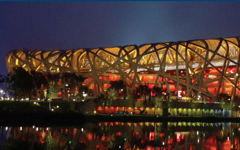
Olympic Sports Complex Beijing, China
