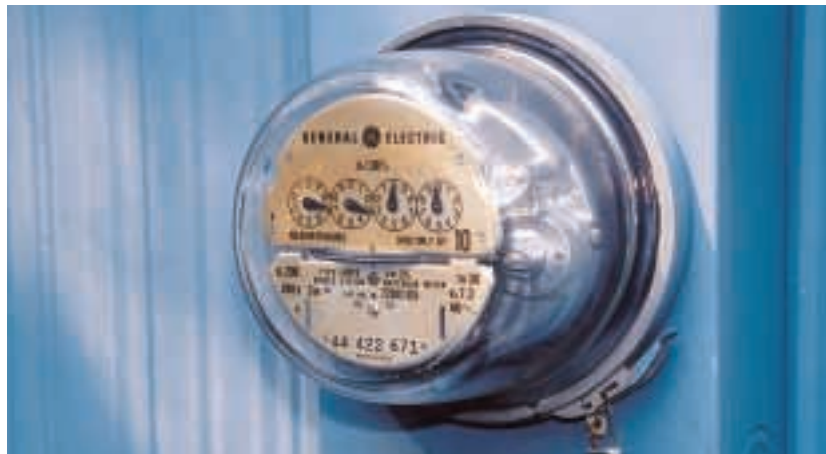
Figure 15.28 The electric meter in your home measures how much energy (in \text{kW} \cdot \text{h} ) that you use.
