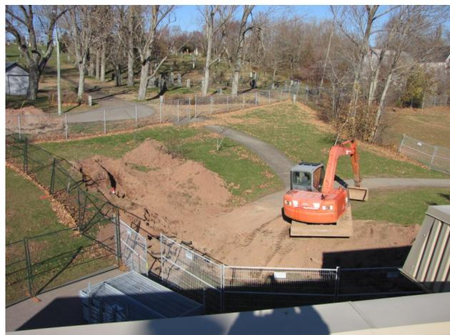
A second project that is being completed by the Town of Sussex is an upgrade of the water line that runs from the school on up through the cemetery. This water line is very old and needs to be replaced. With today's technology the new line will be installed adjacent to the old one using directional drilling technology. This means the only digging is what you see in the picture.
